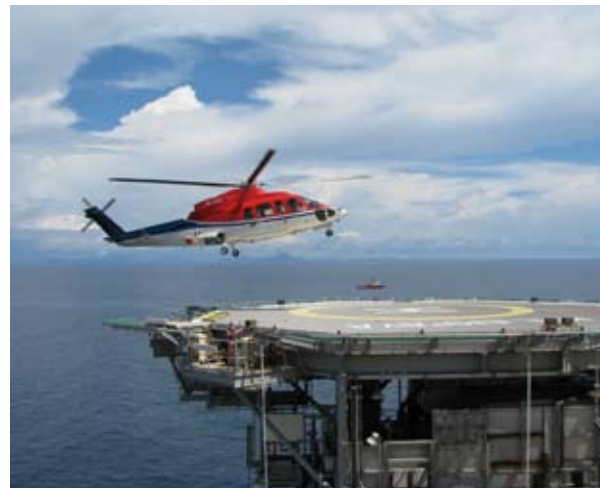
Real-time monitoring of helideck platform
